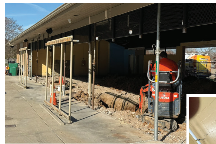
Plumbing roughed in during January 2024.
